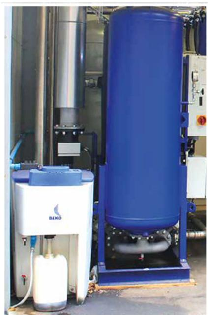
*The installed ÖWAMAT oil-water separator collects and treats the disperse condensate from the customer's compressed air system, independently of the compressor oil.*
