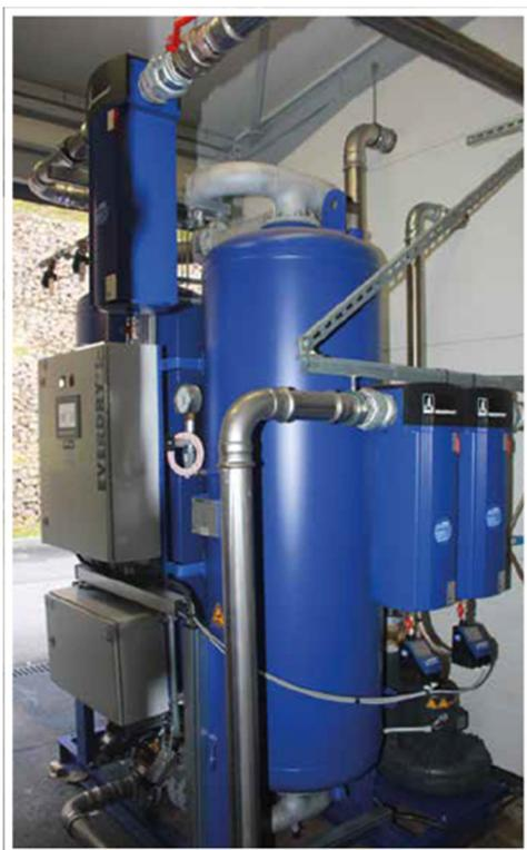
*The heat regenerating adsorption dryer EVERDRY type FRA-V is the heart of the compressed air treatment.*
