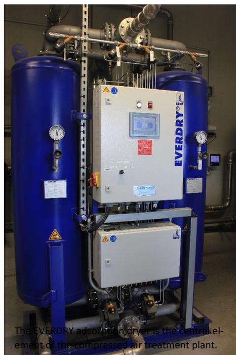
The **EVERDRY** adsorption dryer is the central element of the compressed air treatment plant.
